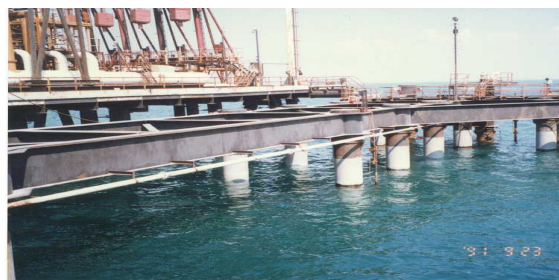
View of some coated piles.
