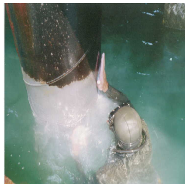
Application by manual spreading of SUBCOM T.260.
