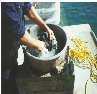
Hand mixing of the 2 components SUBCOM T.260.
