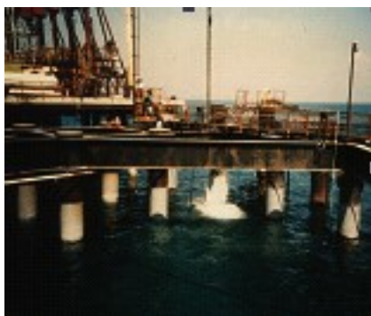
Underwater and splash zone grit-blasting.
