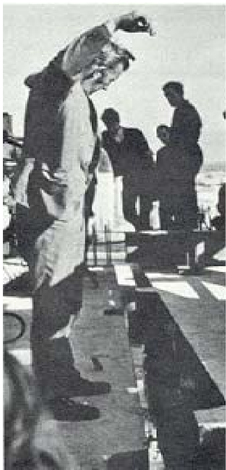
The last few inches as a section is moved into position.
