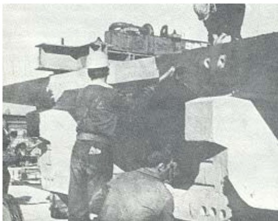
Coating the face of a section with the epoxy adhesive P.A. 103 based adhesive and (right) bringing a closing section between two spans into place.
