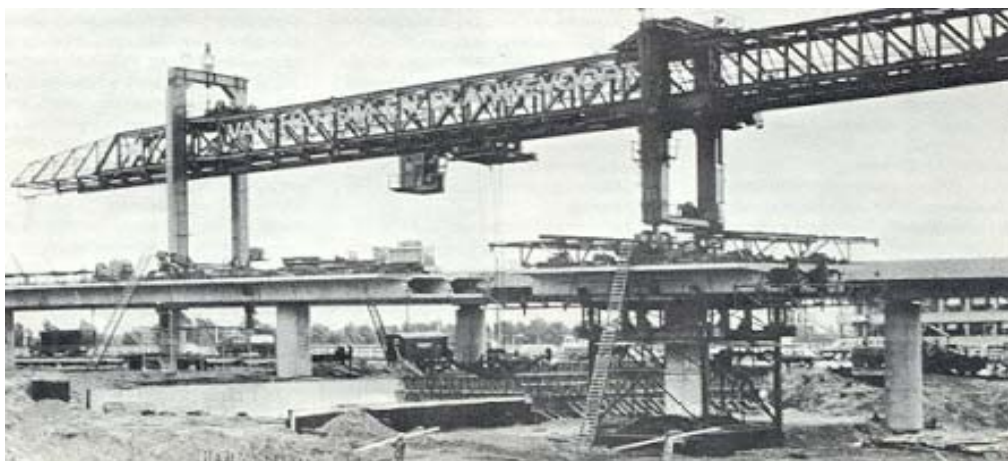
The gantry in position for building a span.
