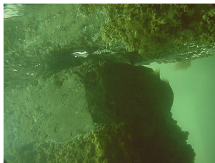
Typical ruptures between concrete piles and platform
