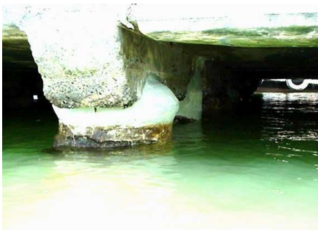
Typical ruptures between concrete piles and platform
