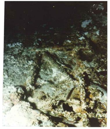
2) Underwater sandblasting of exposed re-bars and concrete
