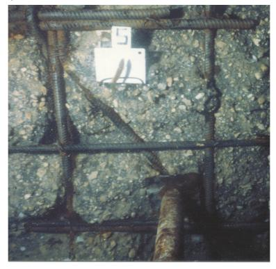
4) Application of SUBCOM T.260 grey color to exposed re-bars and concrete.
