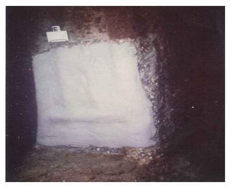
5-6 mm. of SUBCOM T.260 applied on exposed and sandblasted re-bars replace several cm. of Concrete Cover.
