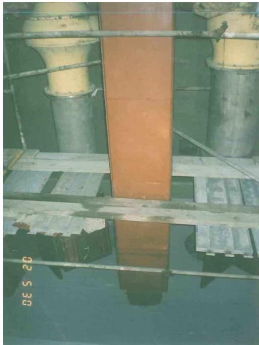
The missing original concrete has been replaced underwater and on wet areas by an epoxy mortar formed by SUBCOM 150 and graded quartz sand, poured in formworks sealed with SUBCOM T.260.
